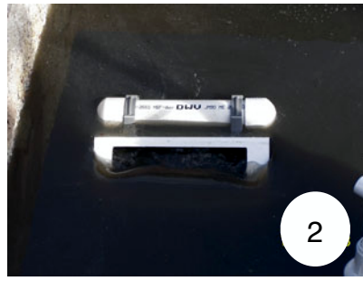
1. The Flout® is free floating, hinging on the flexible connector as the chamber fills. 2 When the Flout reaches maximum, liquid spills in, sinking it and opening the outlet to flow. 3. As the liquid drains down to the top of the Flout, it empties and begins to float again, closing the outlet
