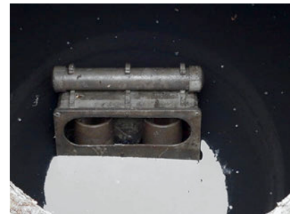
Flout job number 1 in Andover CT. Since 1992, still dosing after all these years.
