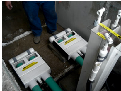
A high flow rate arrangement with two dual 4 inch outlet Flouts and CueBox sequencer
