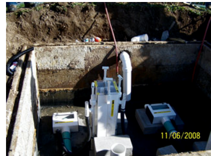
A CueBox™ for sequencing four 28 inch drawdown Flouts.
